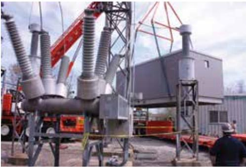
More than 47,000 gallons of dielectric fluid fills the pipe system. The fluid insulates and helps cool the cable during high-load periods. At each end of this pipe-cable system, pressurization plants
